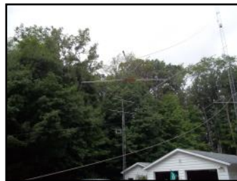
Ground crew has to "balance" the antenna in a sling so it will go up smoothly to the correct face of the tower.
