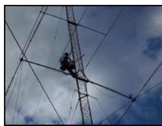
Antenna is trammed into place and secured to the side of the tower
