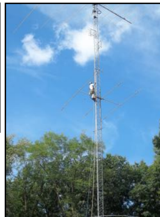
Ground crew has to "balance" the antenna in a sling so it will go up smoothly to the correct face of the tower.
