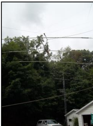
Ground crew has to "balance" the antenna in a sling so it will go up smoothly to the correct face of the tower.
