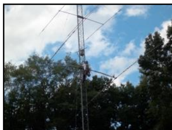
Antenna is trammed into place and secured to the side of the tower
