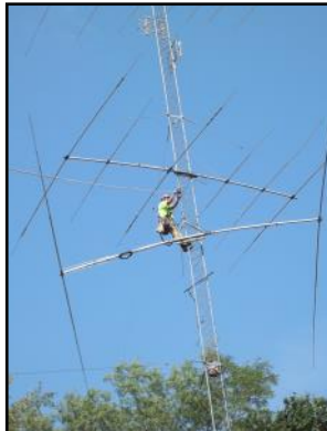
Antenna is lowered on a rope tramline.
