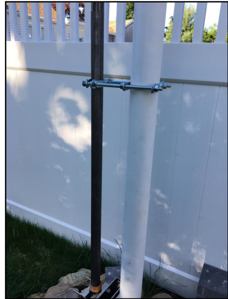
The "clamp" secures the pole to the pipe and reduces sway and weather vaning around the base.
