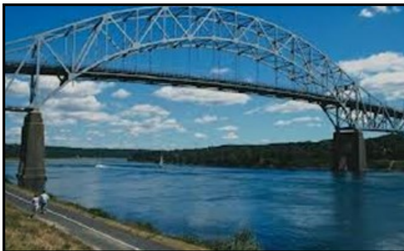
Cape Cod Canal and Bourne Bridge leading onto the Cape.
