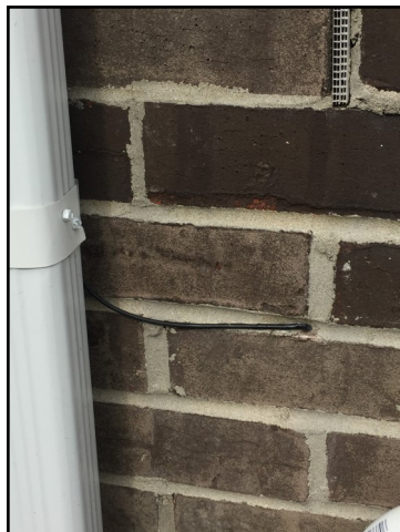
Coax feed through wall
